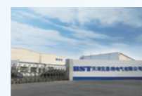
BST factory in Tianjin
